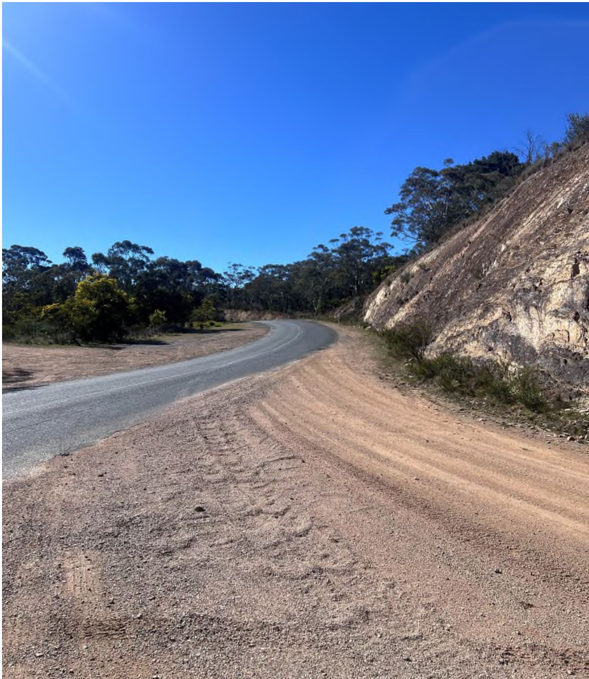
Figure 3: Intersection Cooma Road and Wallaces Gap Road – Existing Approximate Available Sight Distance (looking North)
