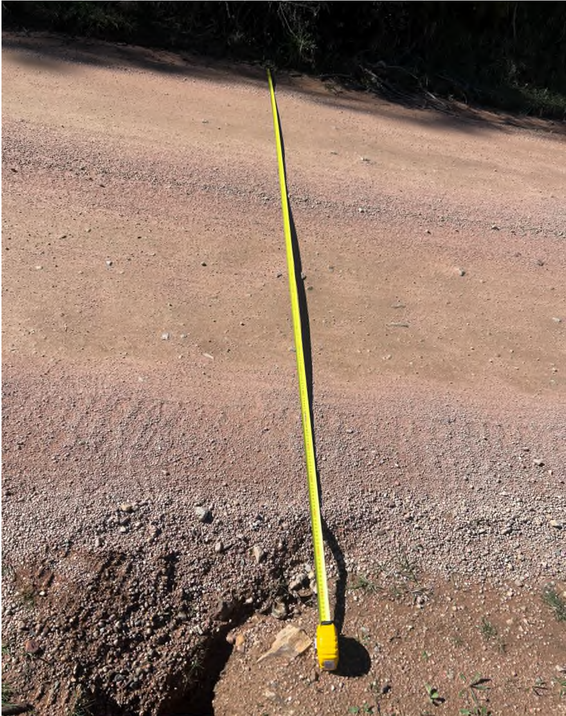
Figure 4: Wallaces Gap Road – Width (3.9m at this section)
